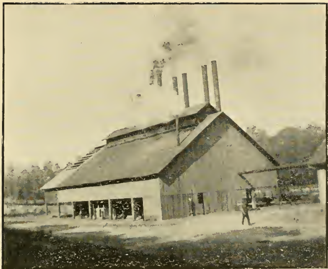
POWER HOUSE AT CONGO MINE.
